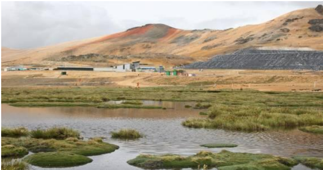
Figure 10 Plant and heap leach, January 2010, showing wetlands in the foreground
